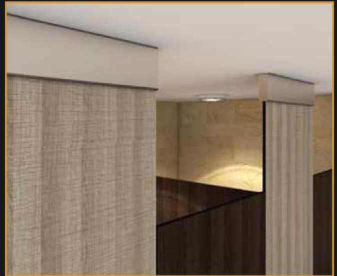
Box up fixtures attached to ceiling
